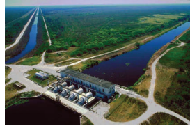
Present-day canals (SFWMD)
