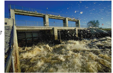
Water management structure releasing water (SFWMD)
