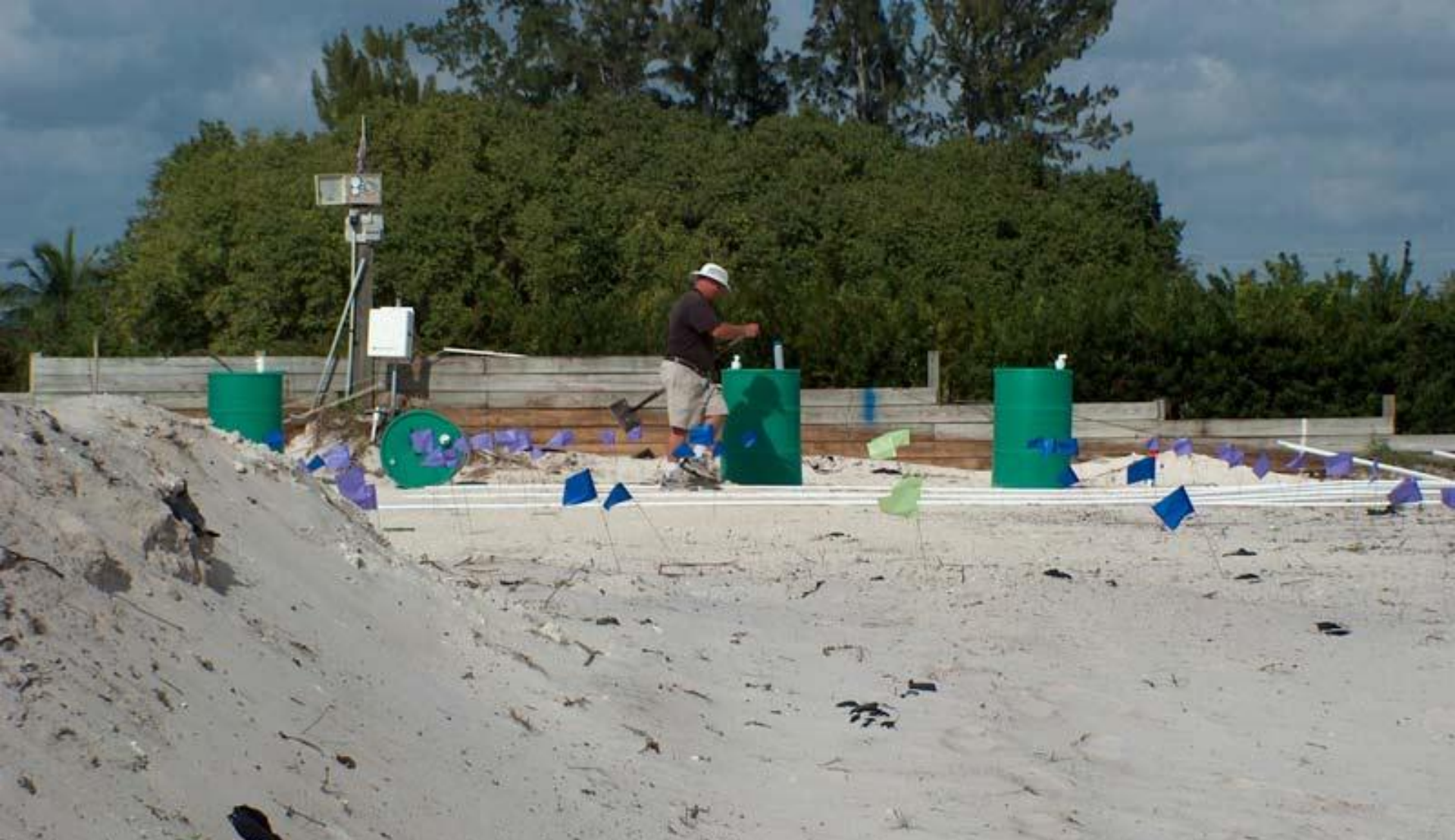
Installation of Lysimeters at Ft. Lauderdale, FL (above grade)
